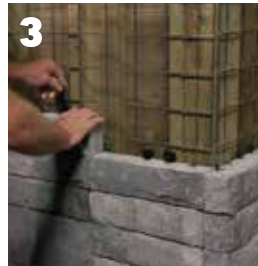
3 Attach Tandem Veneer with Connector
